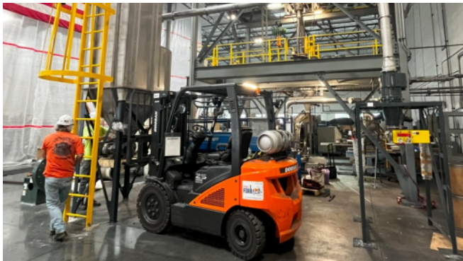
Urbix pilot production facility construction
