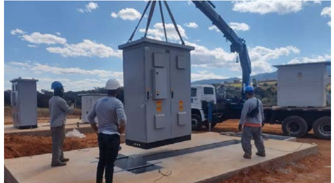
Battery energy storage facility being placed at project site
