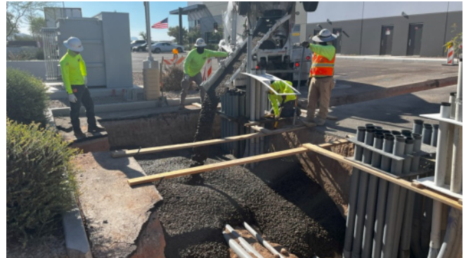
Urbix pilot production facility construction
