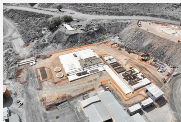
New water treatment plant under construction
