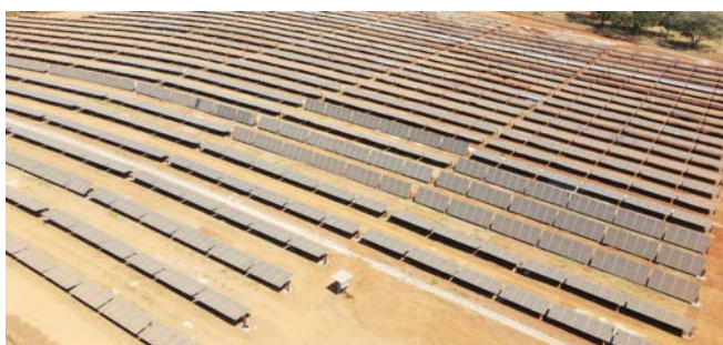
Omnigen solar panels
