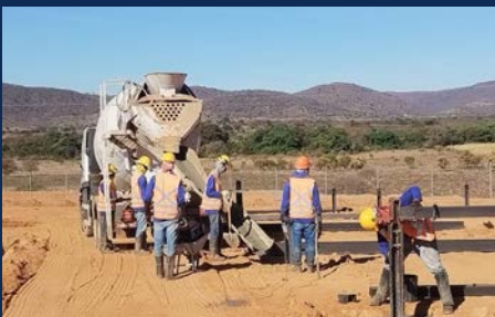
Pouring concrete at the Porterinha site
