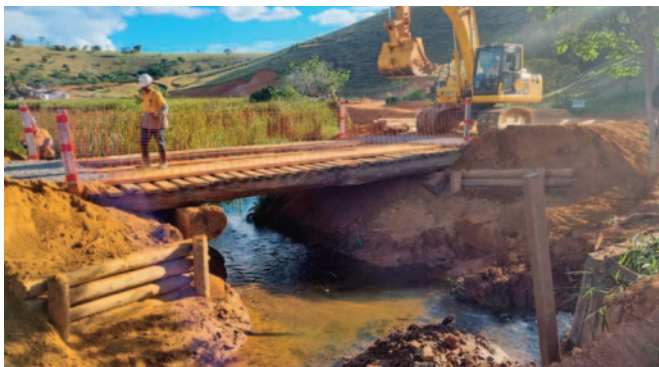
Construction of a bridge to access the site
